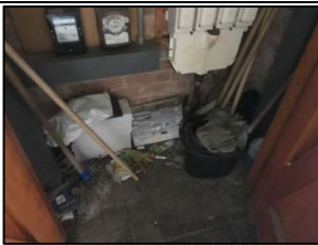
Combustibles in the intake cupboard.
