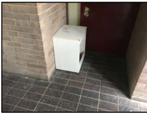
Combustibles in the common area.
