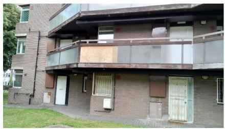
• There is timber cladding between and above windows which is in poor condition
