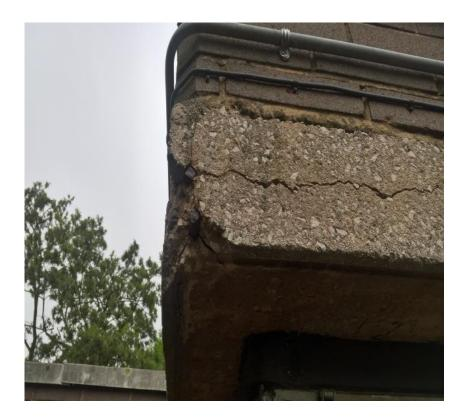
There are a large amount of concrete repairs required to the balcony walkway edges that need to be carried out utilising the scaffolding for Major Works, estimated costs of which would be in the region of a further £1,500,000. A **total budget requirement would be in the region of £10,500,000** for the external and structural works.
