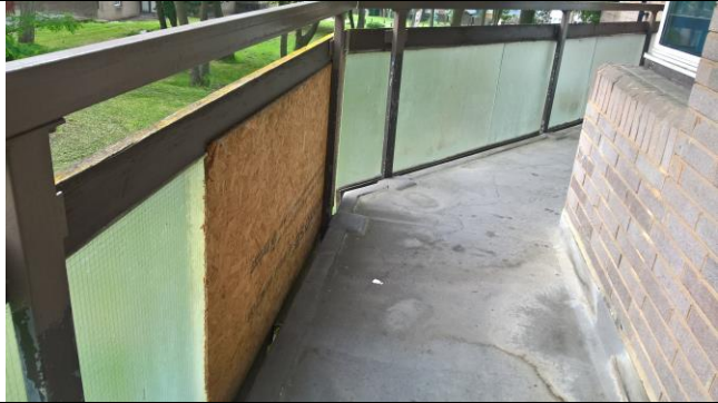
Typical railings to communal balcony (Flats)
