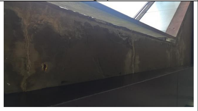
Service duct fixed to the full length of the soffit
