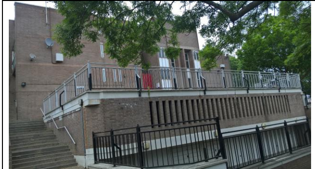
Access stairs to podium & underground garages
