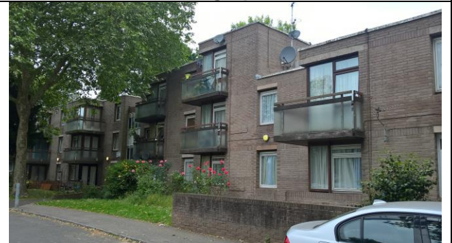
Chalner House –Rear Elevation
