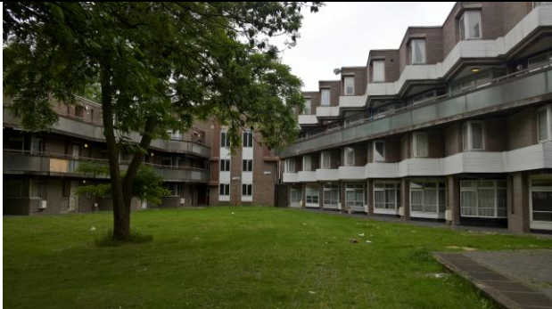
Front elevation of Flats and Maisonettes
