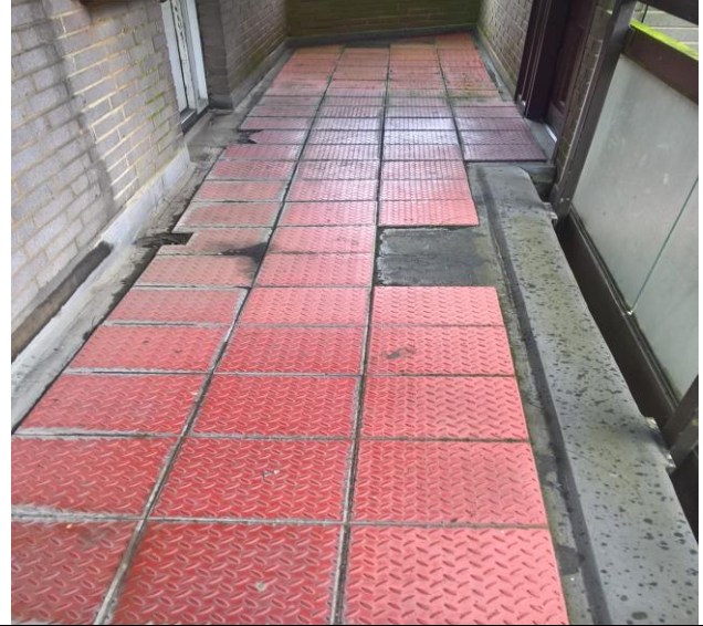
Clay tile laid over old asphalt waterproofing (Despard House Flats & Maisonettes)
